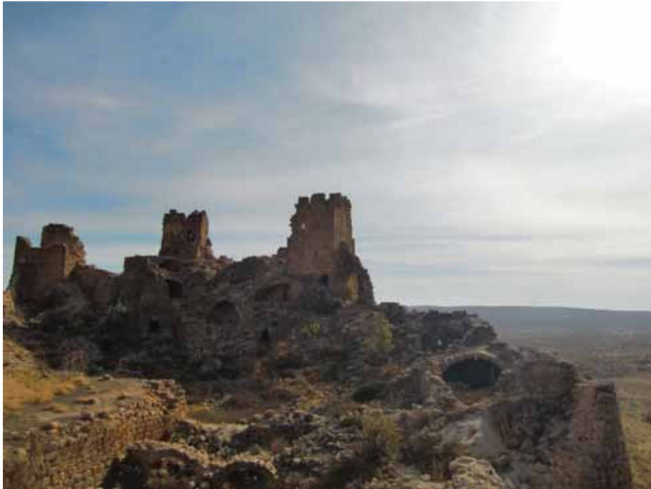
Collapsed monastery of Mor Abhay close to the abandoned village of Beth Man'im. Tradition goes that the monastery had 365 rooms, for each day of the year one. (M. Tozman)
