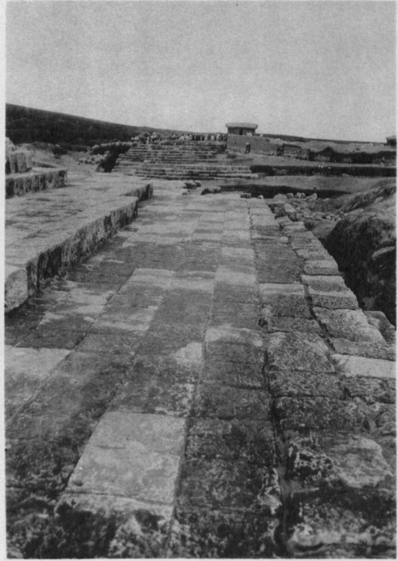
B.—The irregular jointing of the repaired portion (on the right)
