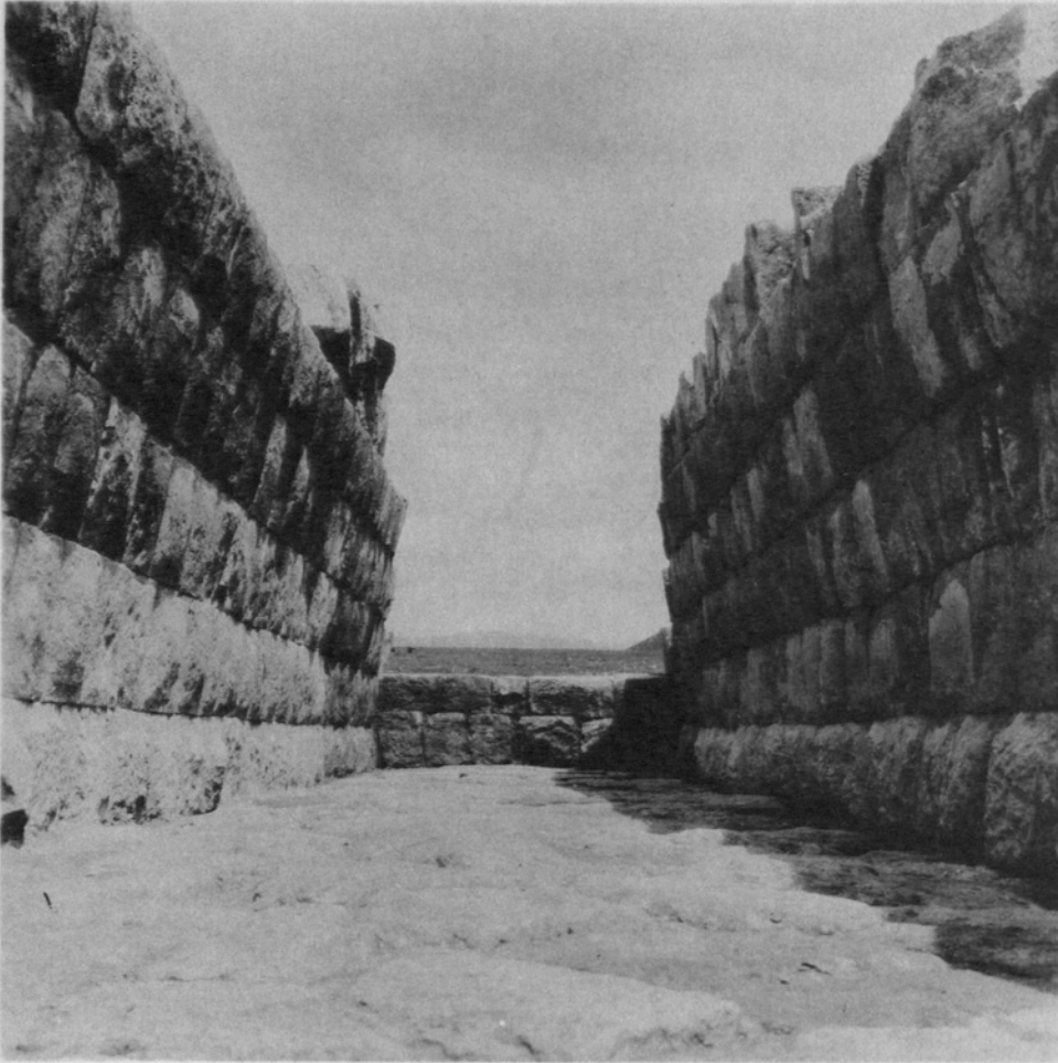
A.—The corbeling of an archway
