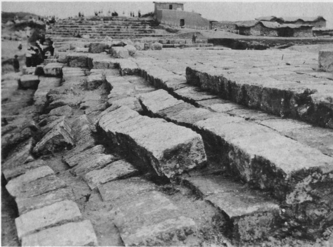
C.—Blocks loosened by settlement
