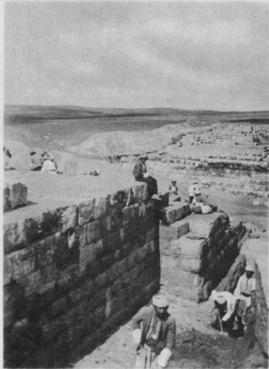
B.—The façade, looking toward the central breach
