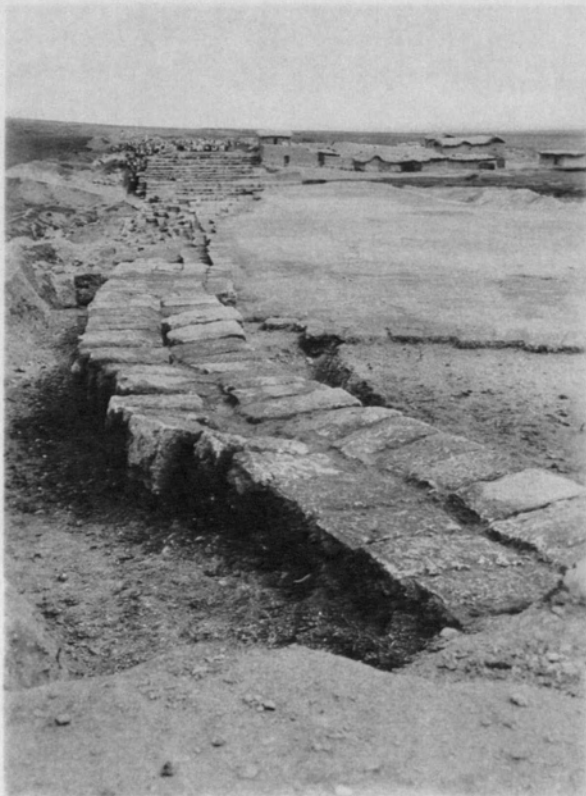
A.—Remains of canal parapet at west end
