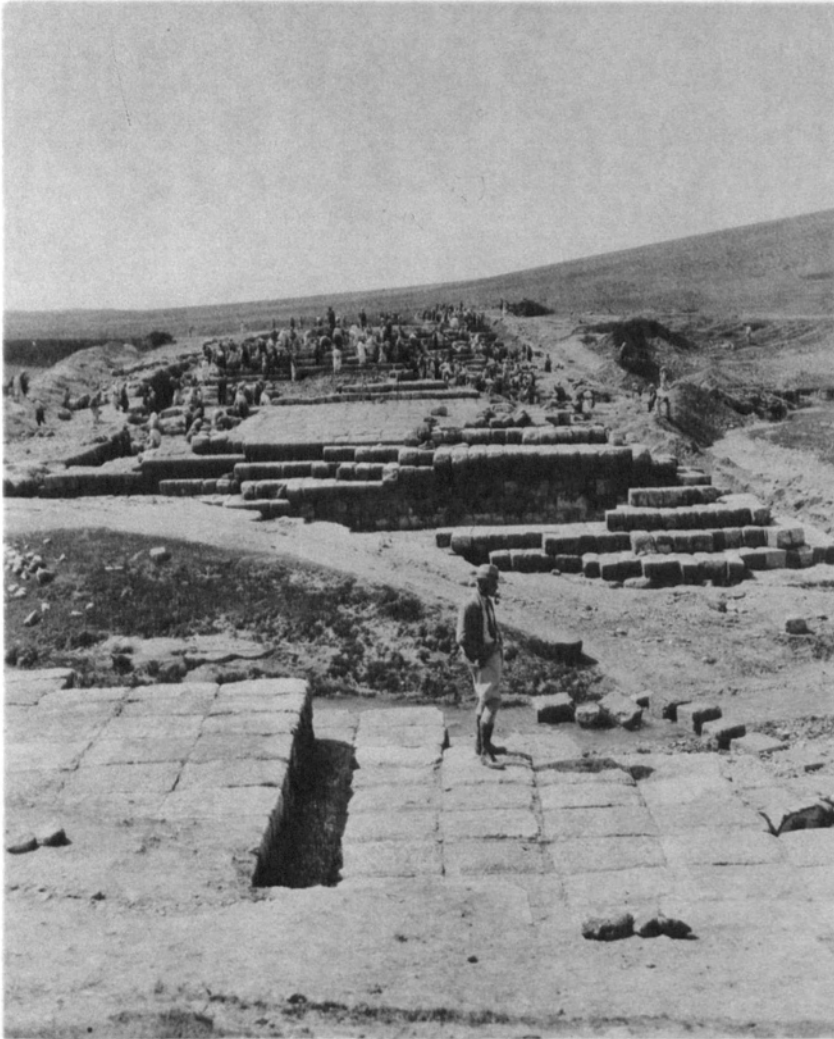
A.—The central breach, seen from the east
