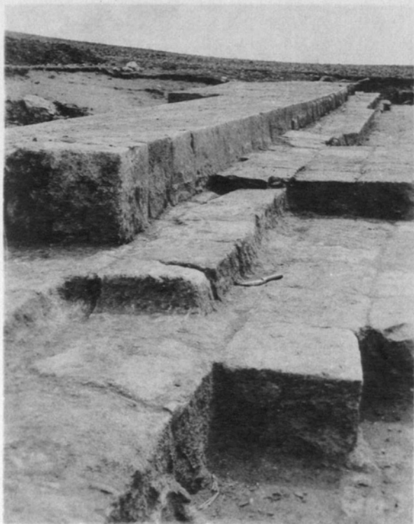
A.—Remains of parapet and paving, showing a few stones of the tilting course
