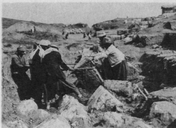
B.—Removal of fallen blocks
