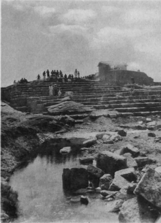
A.—Fallen blocks in the bed of the stream
